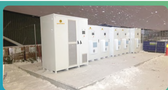
Sweden · All-in-One Solar-Storage-Charging Station with Grid Frequency Regulation Capability Scale:500kW / 1075kWh
