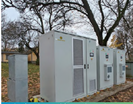
Sweden · Commercial Energy Storage System Providing Grid Frequency Regulation Services Scale:187.5kW / 430kWh
