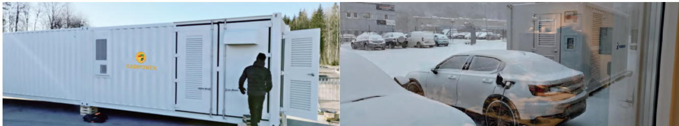
Sweden · Smart Storage-Charging Solution for Workplace EV Charging Scale:500kW / 504kWh
